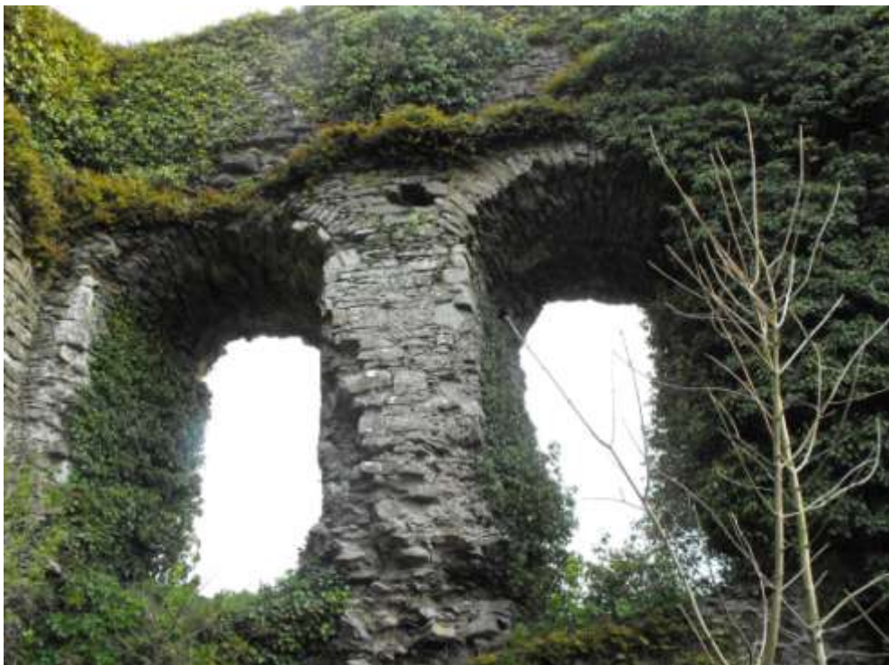
Plate 5.5: Window moulding at Ballyderowen Castle
